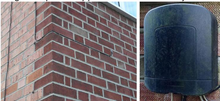
Some properties will have a junction box first, where the external wiring changes into internal wiring. If a single internal wire leaves the junction box then the first socket it reaches is your master socket if multiple wires leaving your junction box this is classed as Star Wiring and BT Openreach no longer support this type of wiring and their call out will be chargeable. Ideally you need a Master Socket upgrade.
