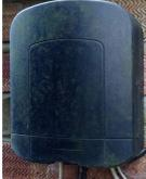
Some properties will have a junction box first, were the external wiring changes into internal wiring. If a single internal wire leaves the junction box then the first socket it reaches is your master socket if multiple wires leaving your junction box this is classed as Star Wiring and BT Openreach no longer support this type of wiring and their call out will be chargeable. Ideally you need a Master Socket upgrade.
