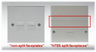
A 'split' type master socket, known as an NTE5, has a horizontal groove in the phone socket and the screws and socket are located in the lower half of the socket. A non-split socket will have the sockets and screws in the middle. You can also identify a split socket looking at the side as bottom half comes out separately.
