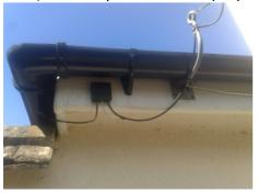
Locate the entry point on the other side of the wall should be your master socket (if you line come out of the ground your entry point will be behind the junction box).
